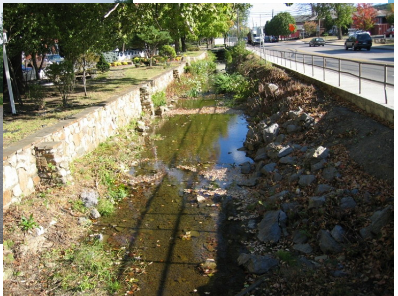
Figure 30: The Run channelized on one side, lined with riprap on the other side
