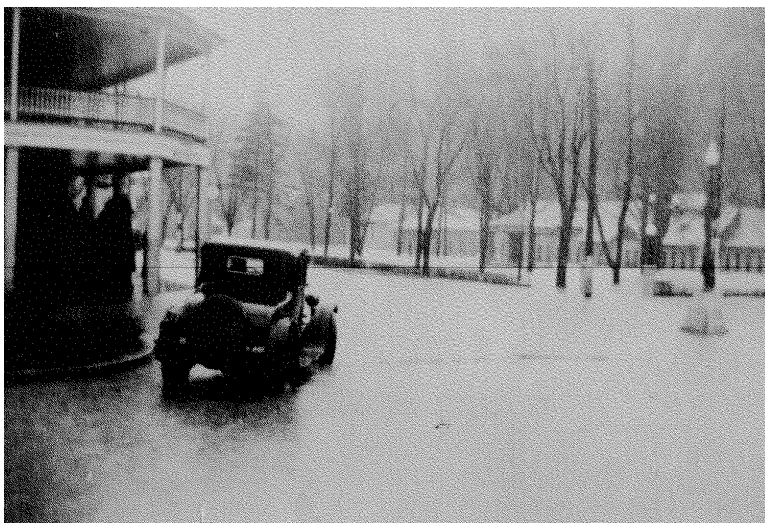
Figure 12: Flooding on Fairfax Street, Berkeley Springs
