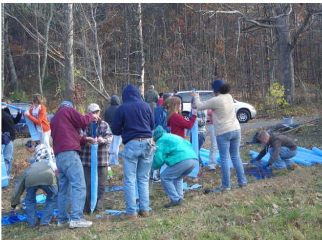
Figure 22 : Repairing the riparian buffer
