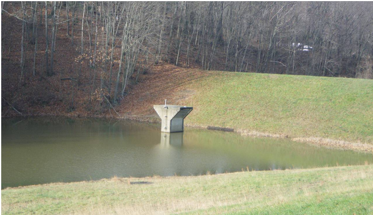
Figure 13: Flood control structure
