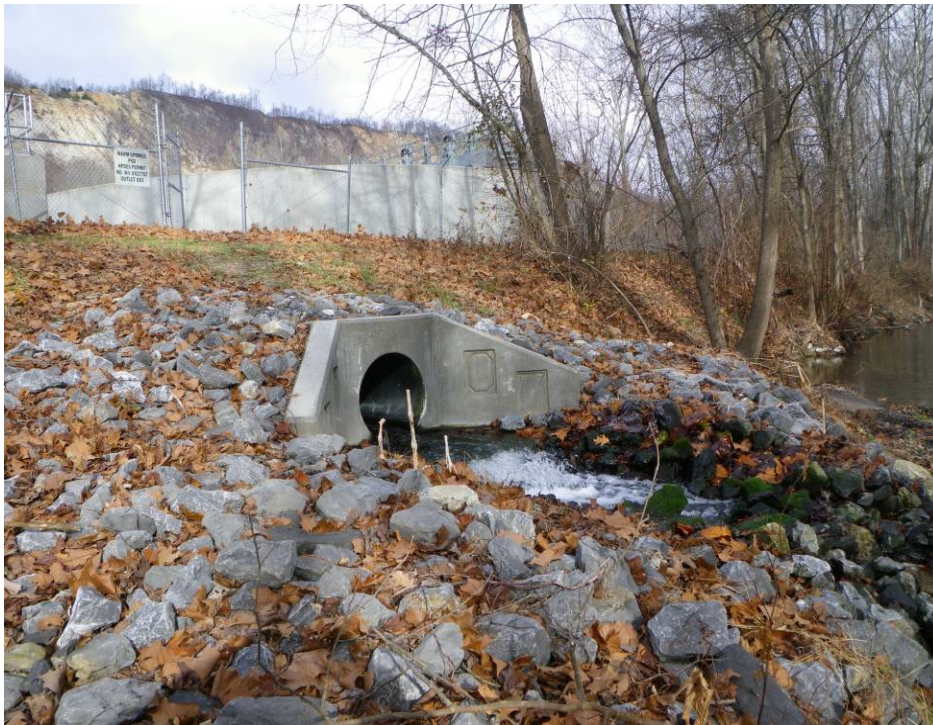
Figure 25: Outfall pipe from the WSPD sewage treatment plant into the Run
