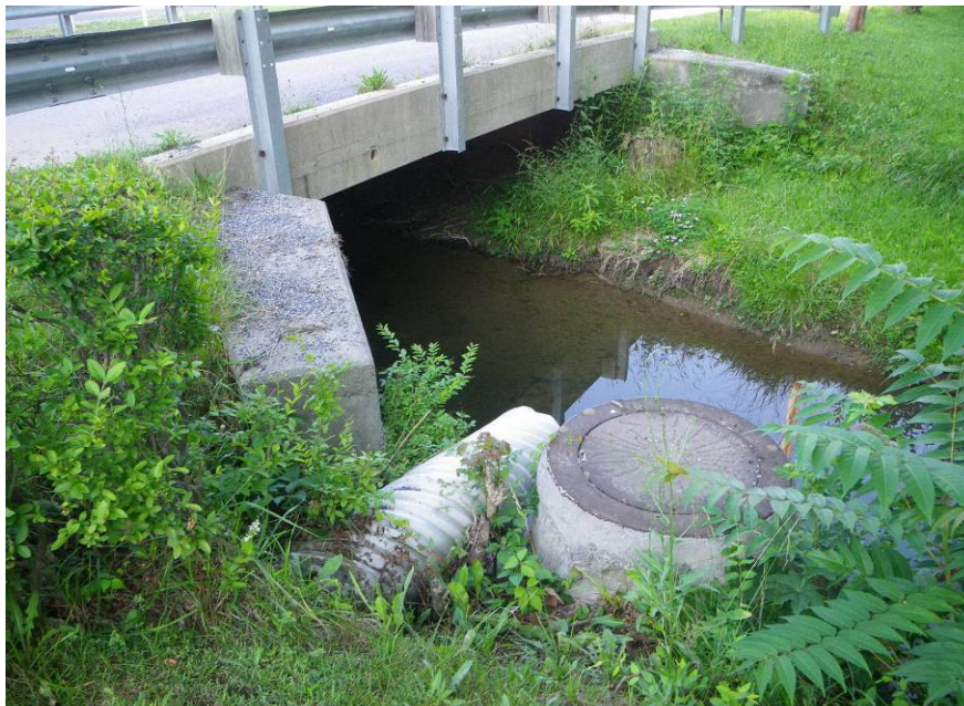
Figure 31: Structures in or near the Run affect its geomorphology
