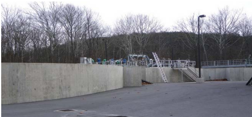
Figure26: Treatment basins at WSPSD wastewater treatment plant
