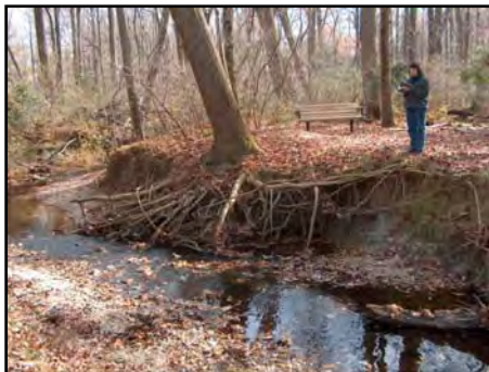
Figure 21 A/B - Snakeden Branch, Reston, VA. Invert raised to reconnect to the floodplain.
