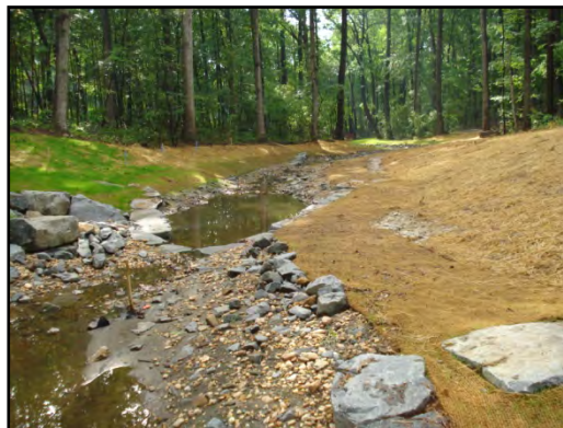
Figure 25 - Snakeden Branch, Reston VA. Newly constructed bankfull bench at lower elevation.
