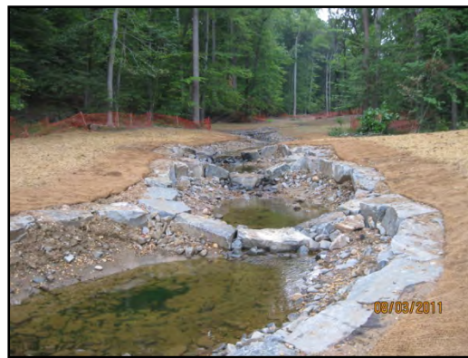
Figure 23 - Fort Belvoir, VA. Newly constructed step pools.
