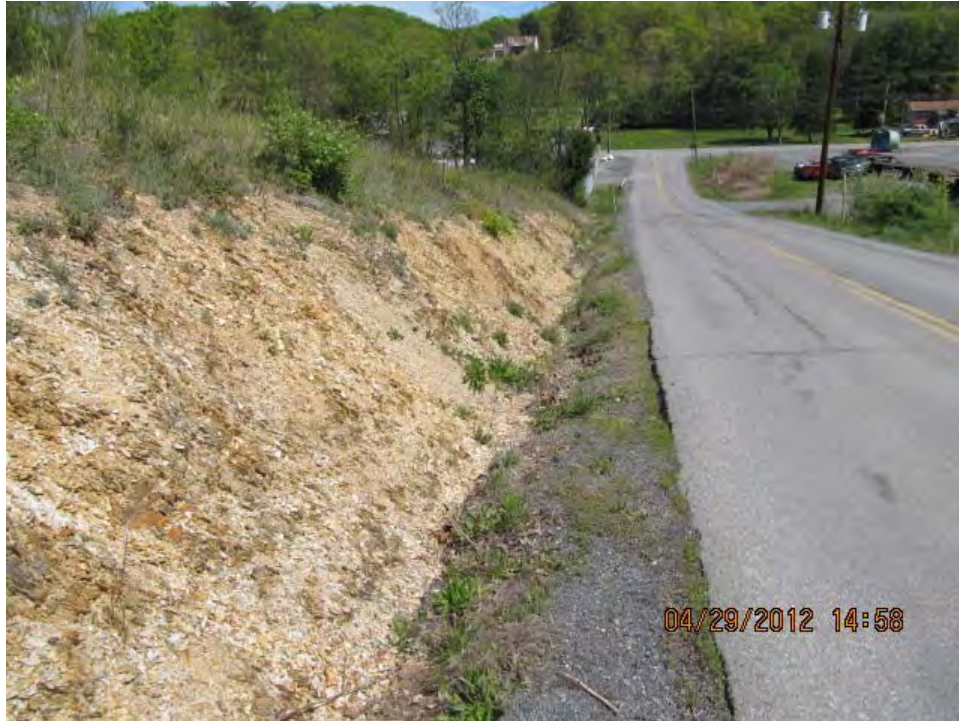
Figure 27. Exposed weathered shale along roadside with minimal vegetative growth after many years.
