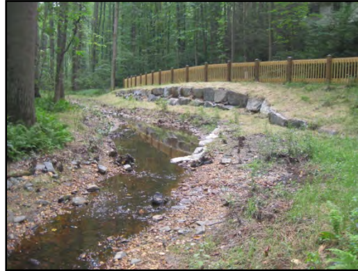
Figure 24 - The Glade, Reston VA. Newly constructed imbricated rock wall to protect trail.
