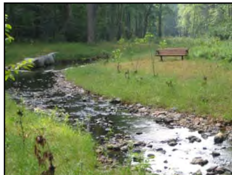
Figure 21 A/B - Snakeden Branch, Reston, VA. Invert raised to reconnect to the floodplain.
