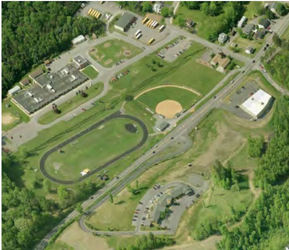
Widmyer Elementary & Commercial Development.
