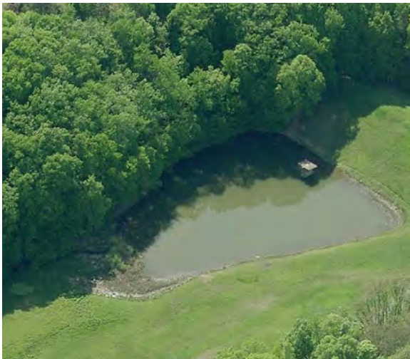
Structure Four Dam and Stormwater Pond. Berkeley Springs, WV.
