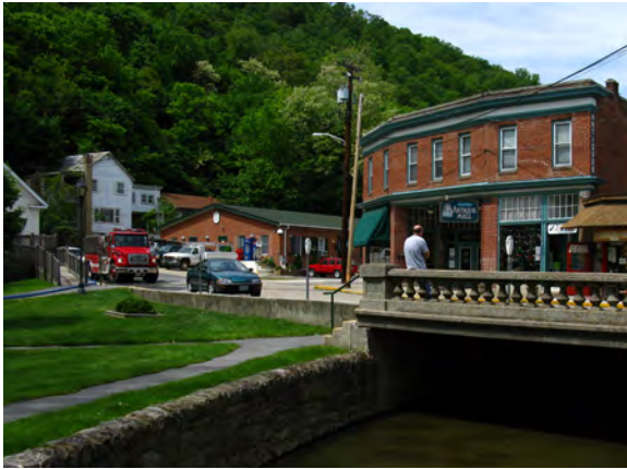
Bridge on Fairfax Street.
