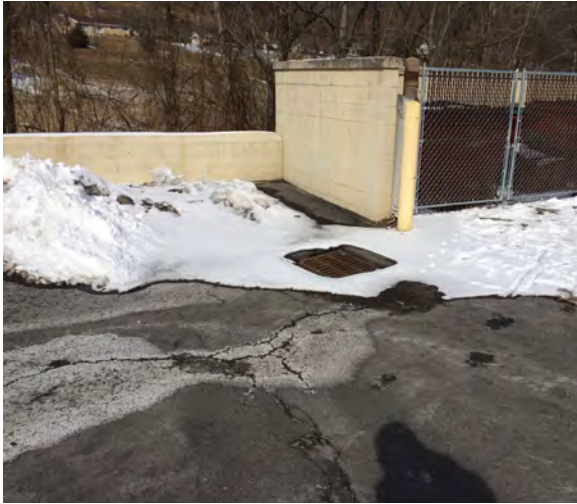
Storm inlet that drains directly into Warm Springs Run.
