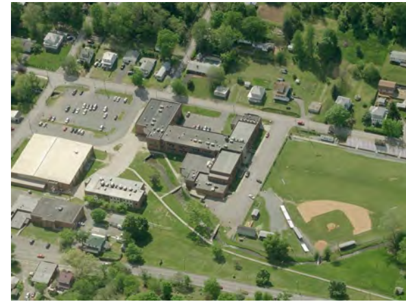
Berkeley Springs High School.
