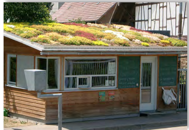
Photo courtesy of www.greenrooftechnology.com
